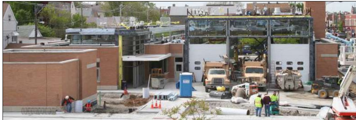
Construction site of the new Engine Company 109.
