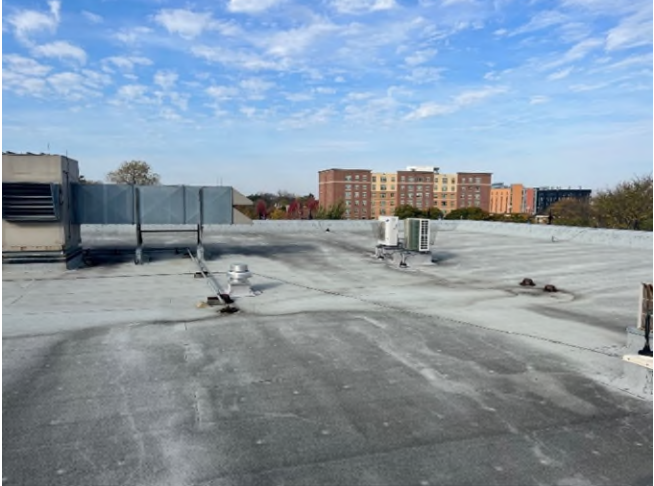
Exist. roof conditions with roof top equipment
