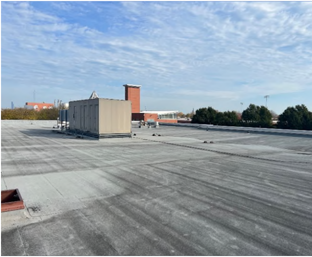
Exist. roof conditions with roof top equipment
