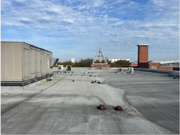
Exist. roof conditions with roof top equipment
