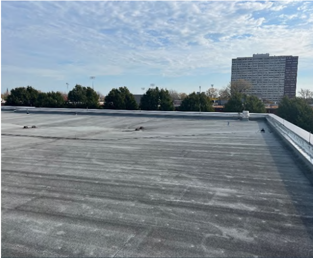
Exist. roof conditions
