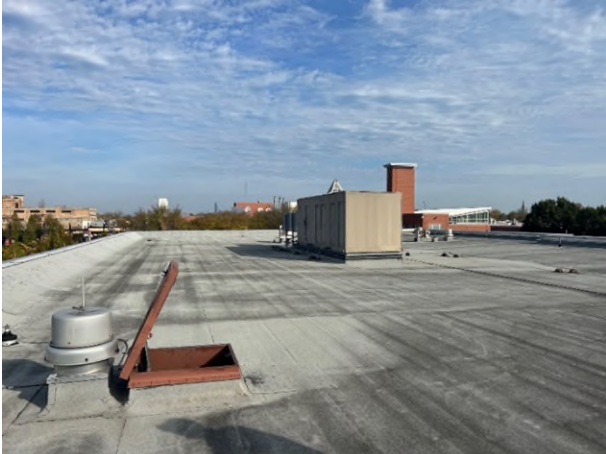
Exist. roof conditions with roof top equipment
