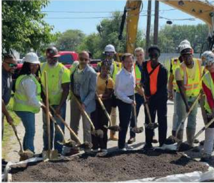
On August 13th, the PBC joined the Chicago Department of Transportation, 15th Ward Alderman Raymond Lopez and community members to commemorate the start of WPA Street Reconstruction: W. 57th Street and W. 58th Street.
