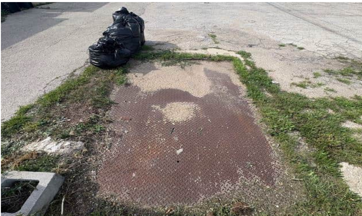
Photo 9 View of a metal vault cover located near the southeast site corner
