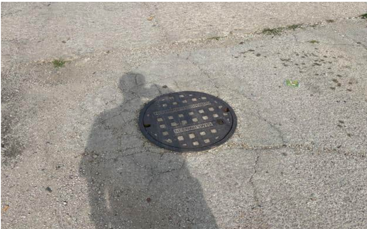
Photo 7 View of a sewer manhole cover located onsite
