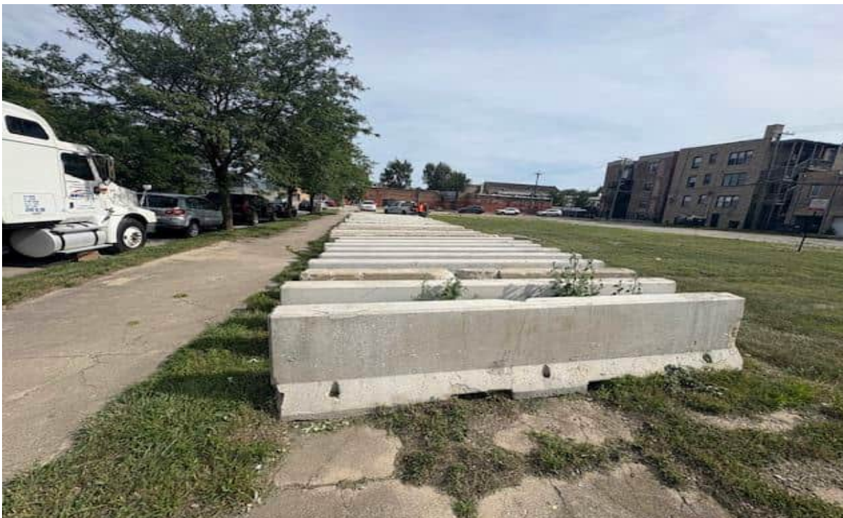
Photo 5 View of concrete barriers located along the western site boundary
