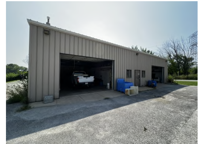
Existing Garage Building
