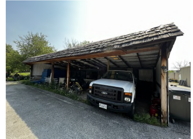
Existing Storage Shed Structure
