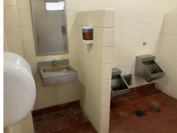
Typical Busse Woods Restroom
