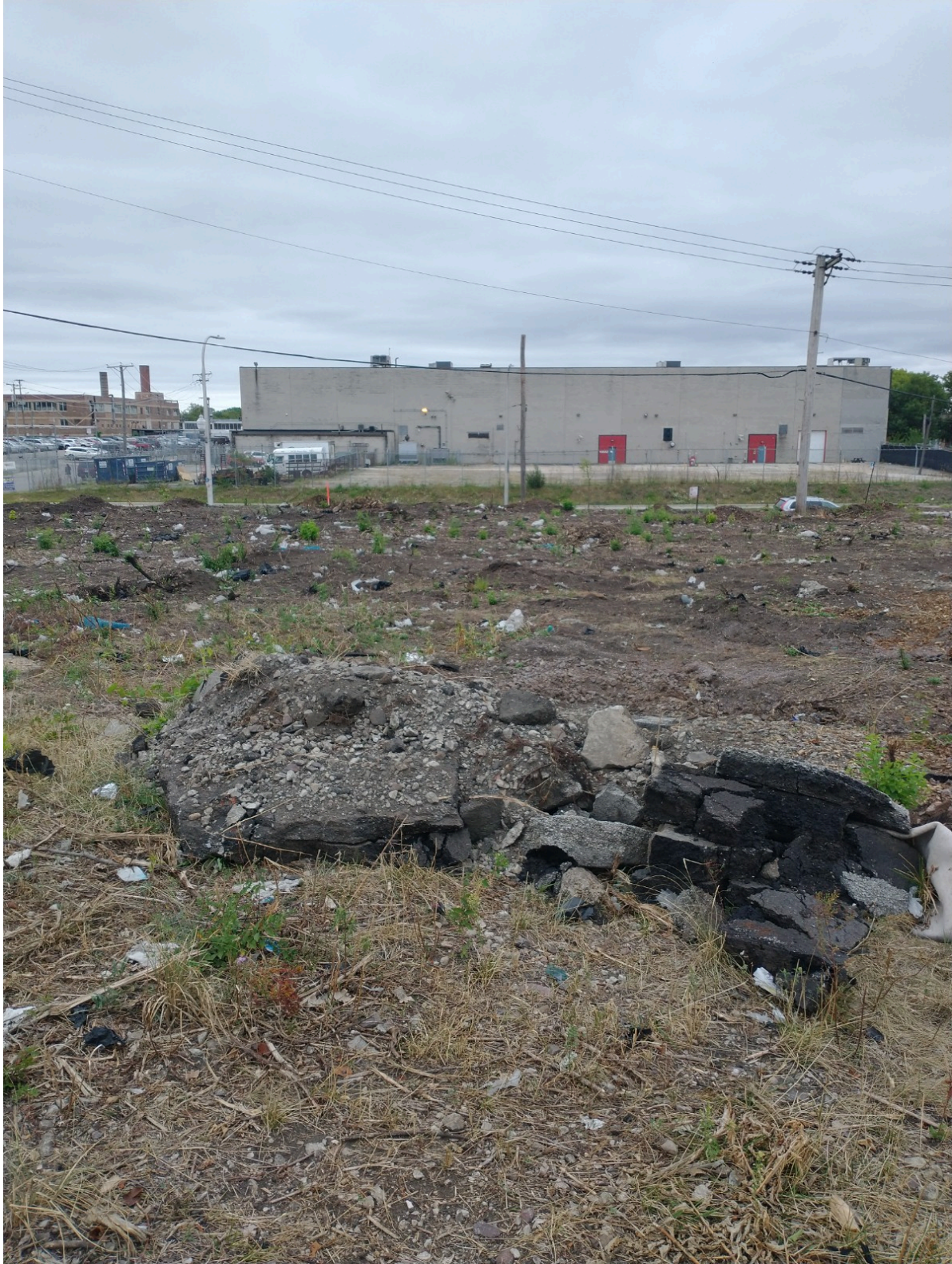
Figure 3 - Photo of site conditions after clearing and mowing
