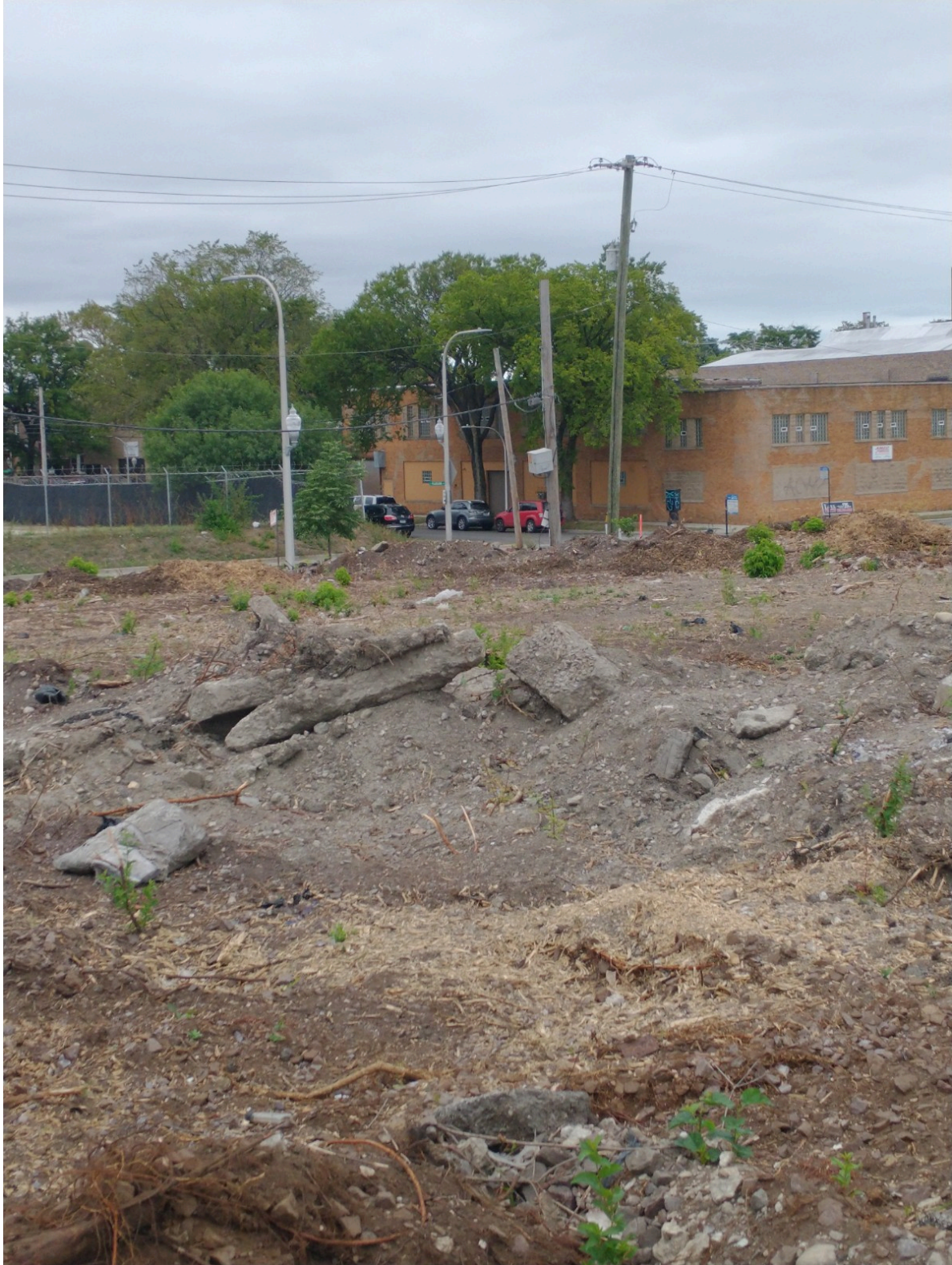
Figure 2 - Photo of site conditions after clearing and mowing
