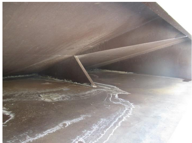
Figure 18. Salt deposits located in the back cavity.
