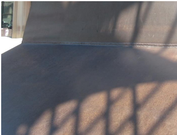
Figure 11. View of cleaned ramped section at south face.
