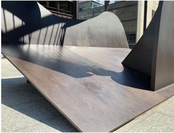
Figure 5. Overall view of the ramped, south facing, portion of the sculpture base.
