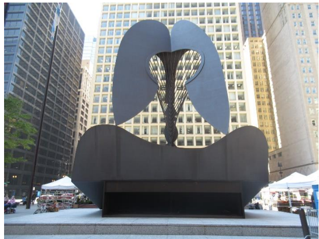
Figure 2. Overall view of the north face.
