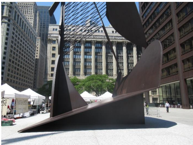
Figure 3. Overall view of the east face.
