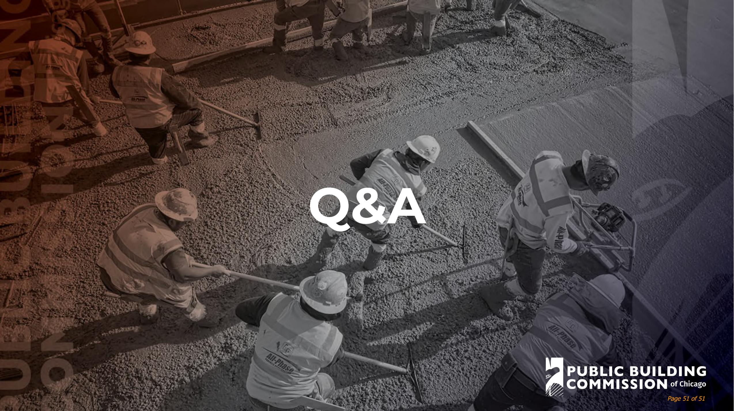
An aerial photograph of a construction site showing several workers in safety gear (hard hats and high-visibility vests) working on a large concrete slab. They are using long-handled tools like screeds and trowels to finish the surface. The scene is captured from a high angle, showing the layout of the slab and the workers' positions. The lighting is bright, casting shadows on the concrete.
