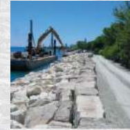
Sloped Stone Revetment
