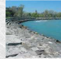
Stepped Stone Revetment
