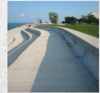
Stepped Concrete Revetment
