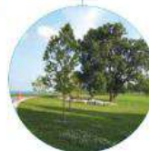
43rd to 45th Street Shoreline Protection, including new laketrail, landscaping and fishing offshore reefs
