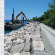
Sloped Stone Revetment
