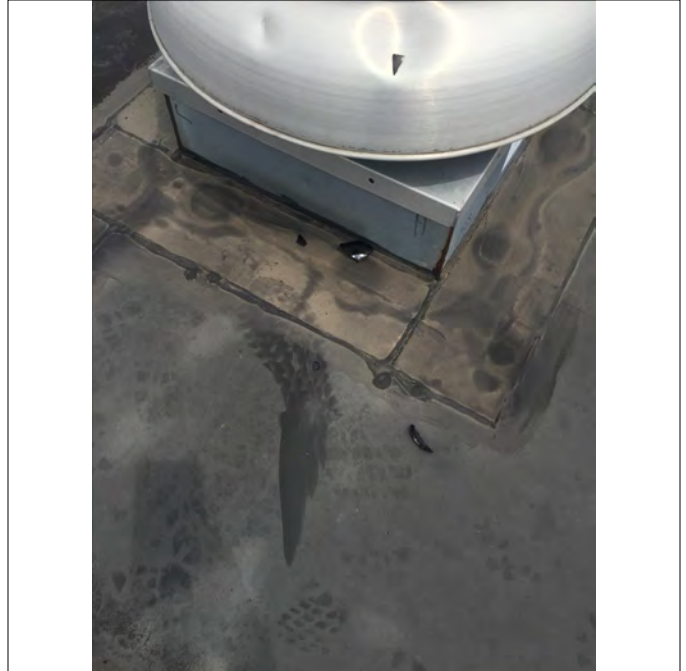
HOLE IN MEMBRANE
