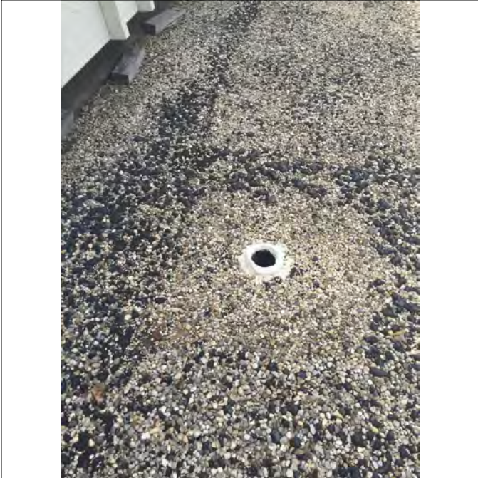
LOW ELEVATION OF FLASHING
