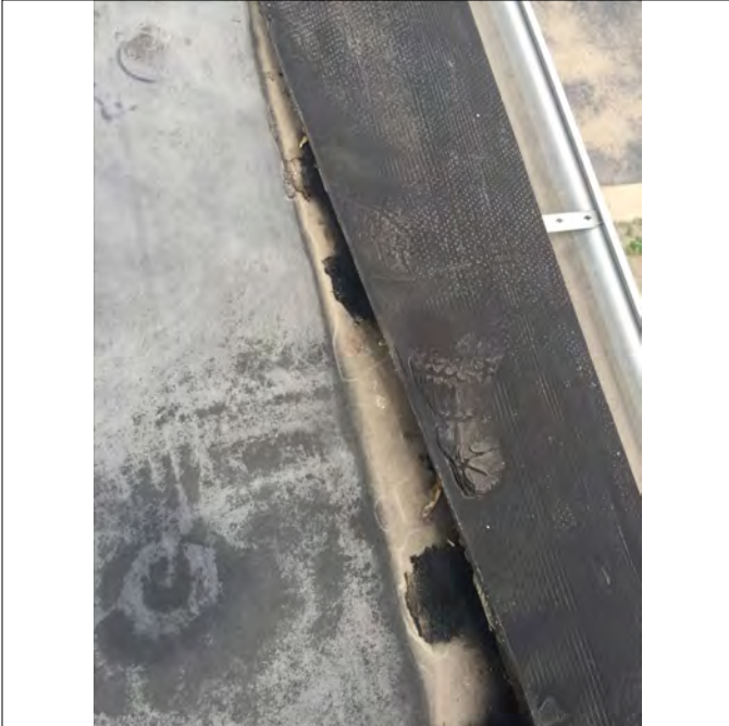
LOOSE MEMBRANE REPAIR
