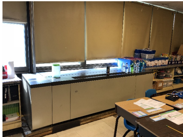
Photo 21 View inside classroom 130. Note the encased fan coil unit with poor installation condition. The wall insulation adjacent to unit is torn apart causing weather tightness issues around the year.
