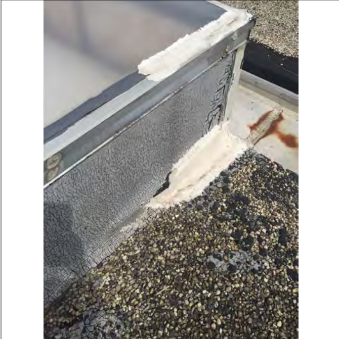
LOOSE FLASHING
