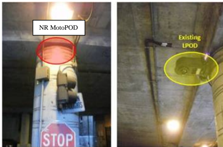
Figure 6—New NR MotoPOD Location Figure 7—Existing LPOD
