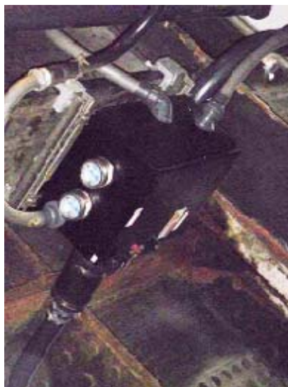
Figure 4—Existing MPOD and JPOD power on the southwest corner of Lower South Water and Columbus
