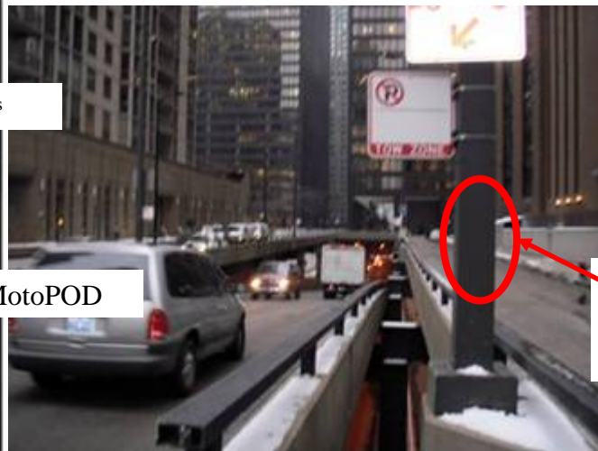
Figure 3—View from mounting location towards Lower Wacker Entrance / Exit
