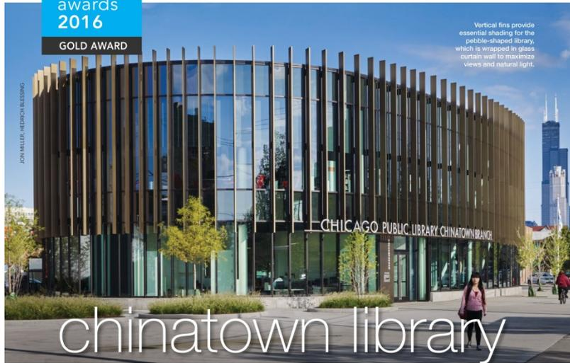
Vertical fins provide essential shading for the pebble-shaped library, which is wrapped in glass curtain wall to maximize views and natural light.
