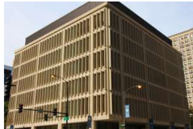
WILLIAM JONES COLLEGE PREPARATORY HIGH SCHOOL RENOVATION 606 South State Street Ward 2
