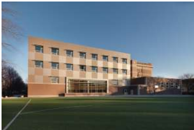
JOHN C. COONLEY ELEMENTARY SCHOOL ADDITION 4046 North Leavitt Street Ward 47
