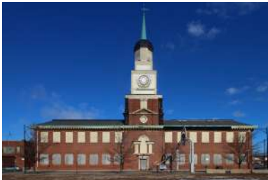
STOCKYARDS BANK STABILIZATION 4146 South Halsted Street Ward 11
