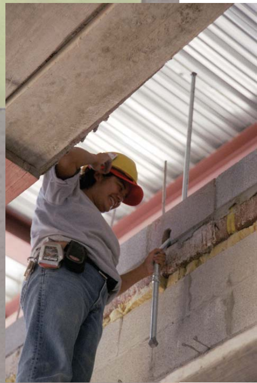
8th District Police Station under construction
