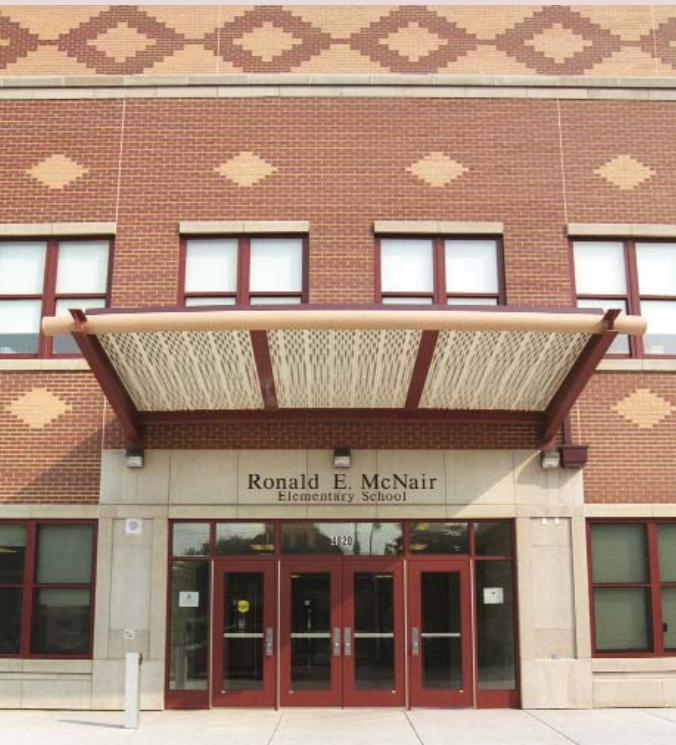
Ronald E. McNair Elementary School façade
