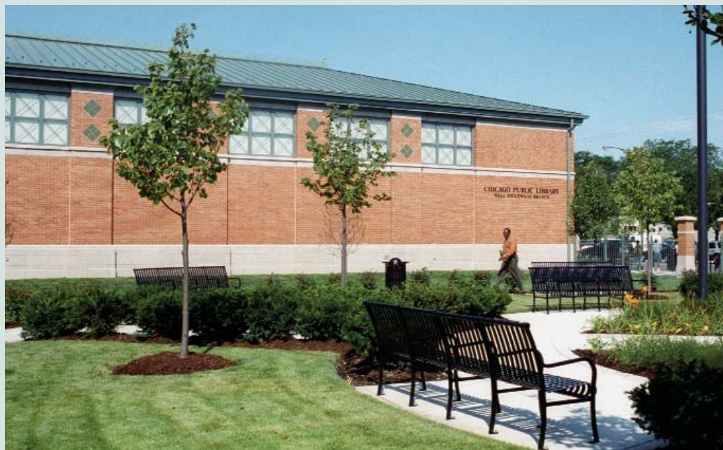
The new West Englewood Branch Library
