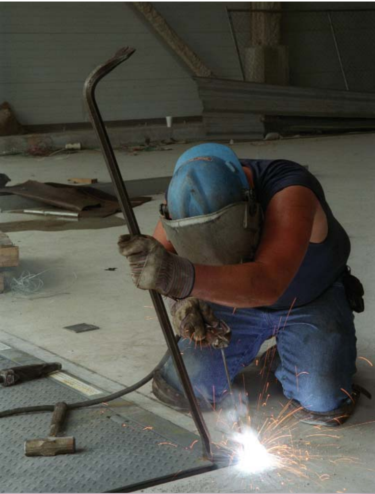
Welding at the construction site of the Department of Water Facility
