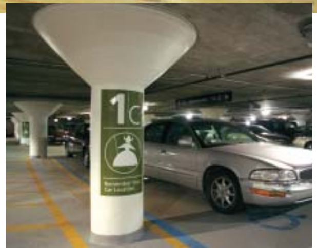
Grant Park South underground parking
