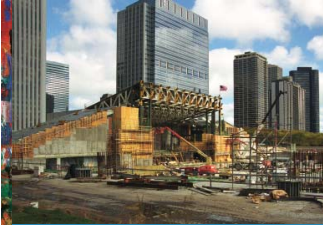
Gebry band shell under construction
