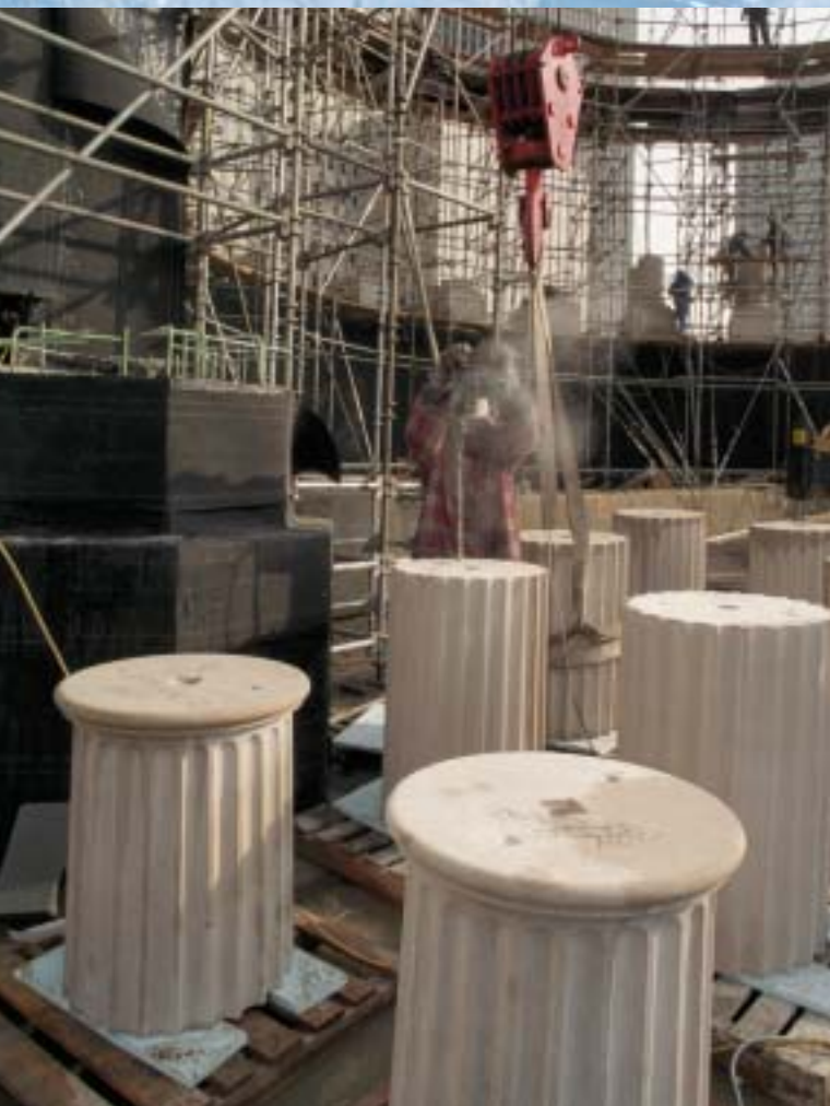
Millennium Park Peristyle under construction
