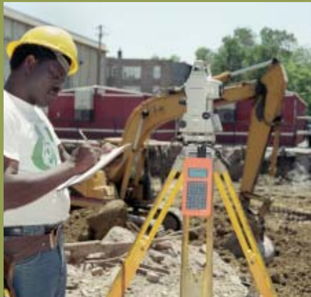
Pre-construction activity at the future site of the Edward "Duke" Ellington School
