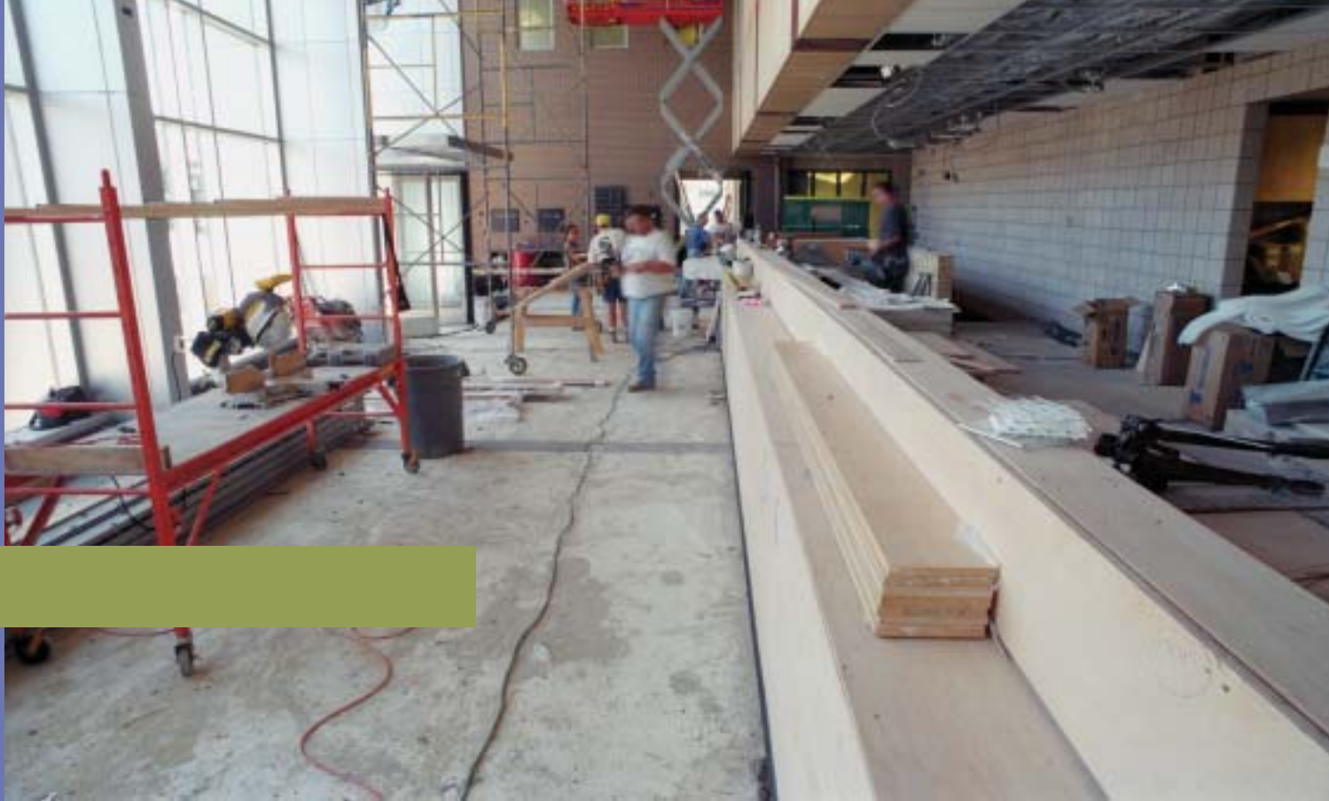
Interior construction at 20th District
