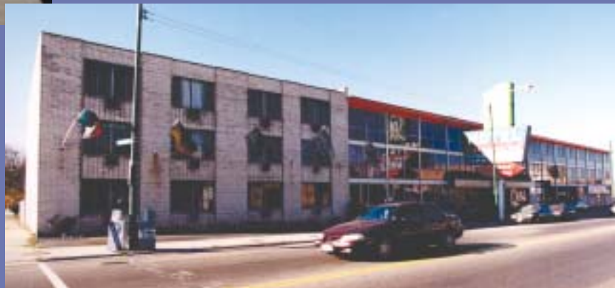
The former Spa Motel at site of new 20th District Police Station
