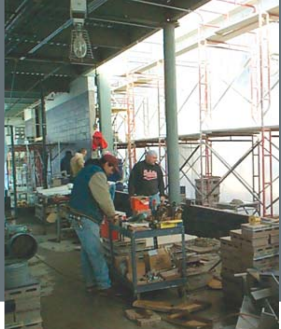
Construction at Hayes Park Natatorium
