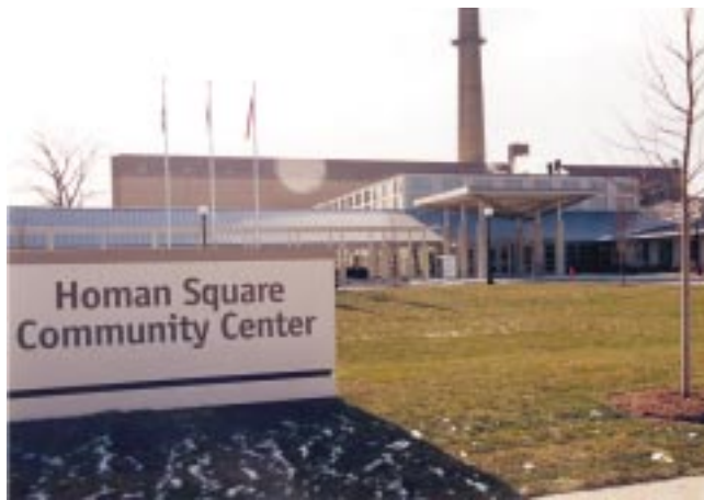
Photos: (top & at left) Grant Park South construction activity; (Center) Hawthorne Park Family Entertainment Center architectural illustration; (bottom) Homan Square Community Center & Fieldhouse
