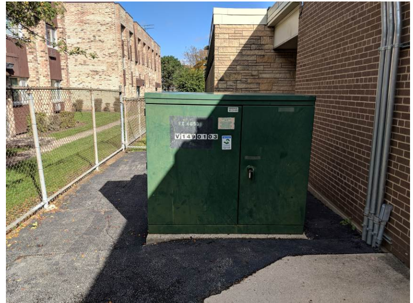
Photograph 12: Pad-mounted transformer located on the west side of the main structure.
