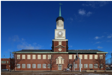
STOCKYARDS BANK STABILIZATION 4146 South Halsted Street Ward 11
